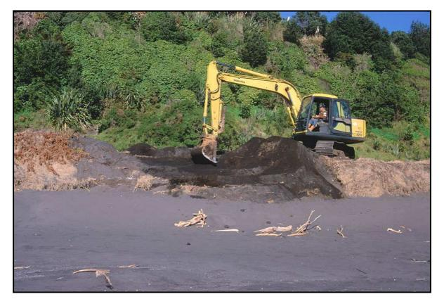
Figure 6: Sand was taken from near high water mark and moved landward. Where practical, consolidated layers of clay or other compacted fill were placed towards the back of the dune.
