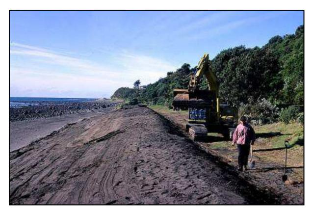
Figure 8: The final stage of mechanical reshaping involved smoothing off the dune to a 15° slope for the planting of sand-binders. Care was taken to ensure the toe of the newly reshaped foredune did not extend beyond the position of high water mark before reshaping.
