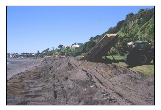
Figure 7: Sand was shifted from the eastern end of the trial site where there was a surplus to the western end to make up for a deficit of material required to form a reshaped dune.
